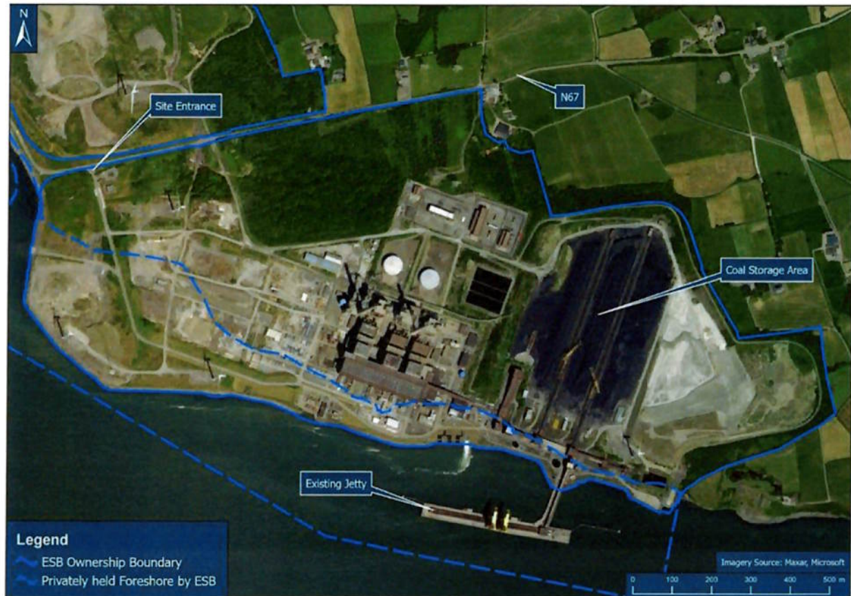
Figure 1.1: Moneypoint Generation Station, ESB Landownership Boundary
